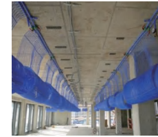
结构面抹灰 Structural Plastering
